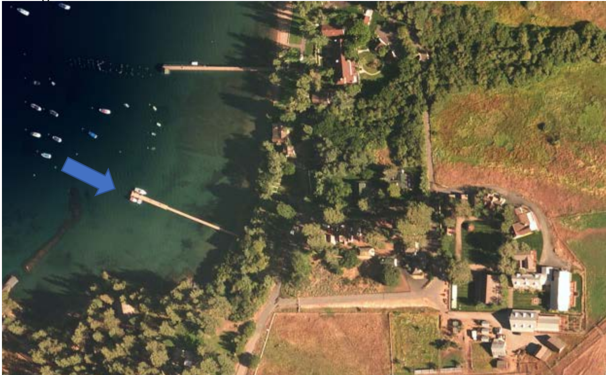
Existing Pier without Extension
